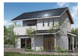
Tokyo Sekisui Heim Co., Ltd. Enlarging the roof to increase PV capacity
