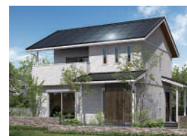
Tokyo Sekisui Heim Co., Ltd. Enlarging the roof to increase PV capacity
