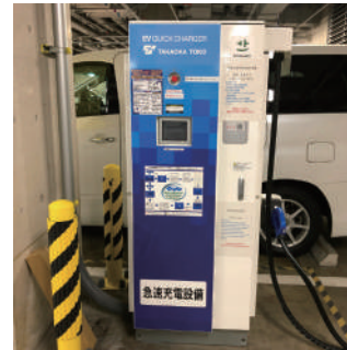
Fast charger with 50-kW output
