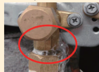
Leakage of fluorocarbons
