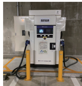
Fast charger with 90-kW output (2-port type)
