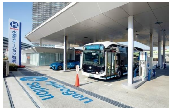
Bus-capable Hydrogen Station
