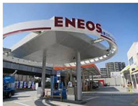
Hydrogen station utilizing a TMG-related site (Dr. Drive Self Shiomi Park SS)
