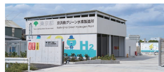
TMG Keihinjima Green Hydrogen Plant
