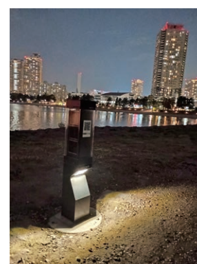
Initial introduction to TMG facilities A garden light in Odaiba Marine Park
