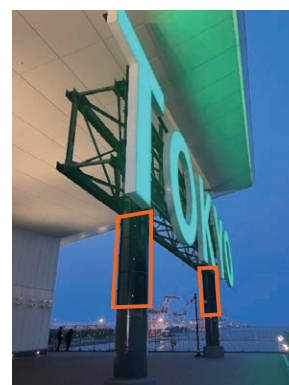
Air Solar installed on the pillars at a port facility
