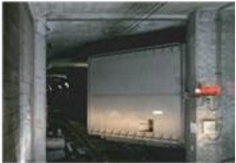
Waterproof gate in tunnel
