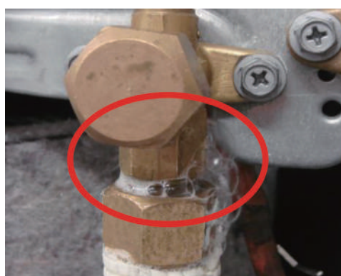
Leakage of fluorocarbons
