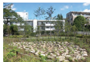
Rain Garden in Setagaya Ward where rainwater in the vicinity is collected and infiltrated underground
